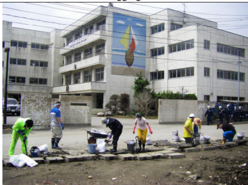
側溝泥だし 3 Digging mud and debris
