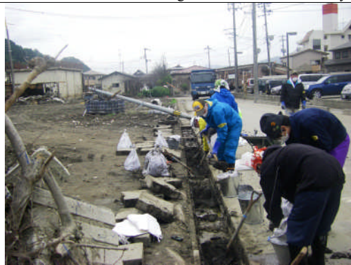
側溝泥だし 1 Digging mud and debris
