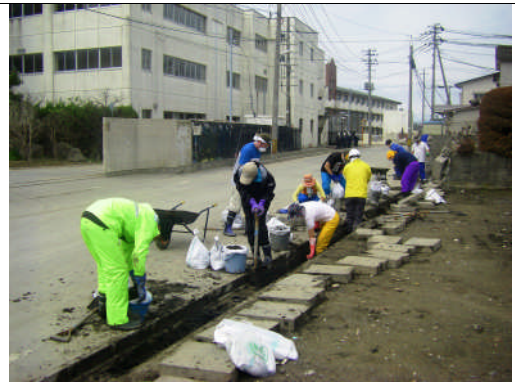
側溝泥だし 2 Digging mud and debris
