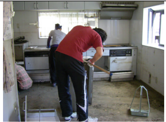
泥だし 2 Clear debris
