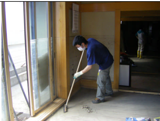
泥だし 3 Clear debris
