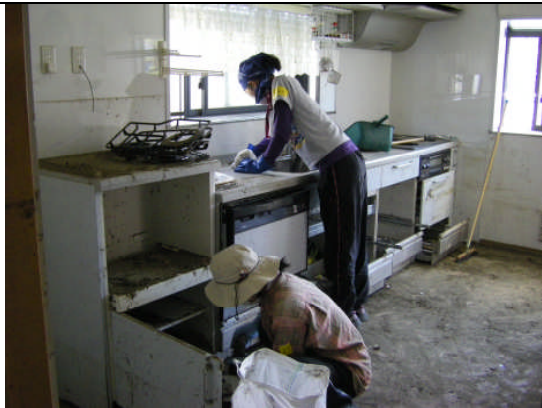
泥だし 1 Clear debris
