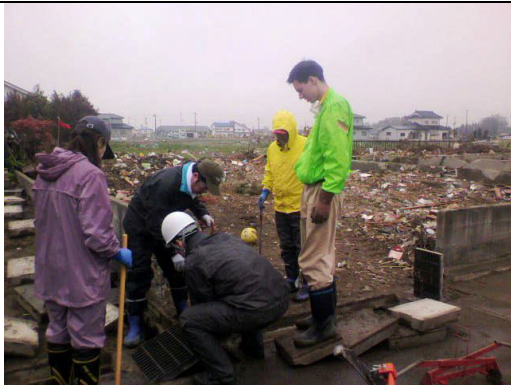
Removing lids 側溝の蓋はずし
