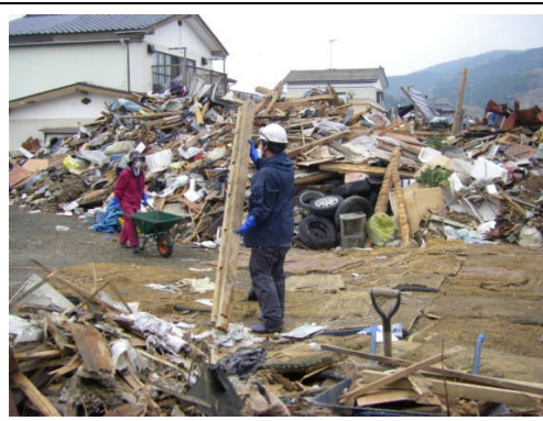
Debris cleaning up at Myojinsha
