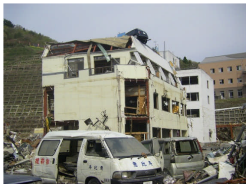
Tsunami attacked 4 th floor of buildings.
